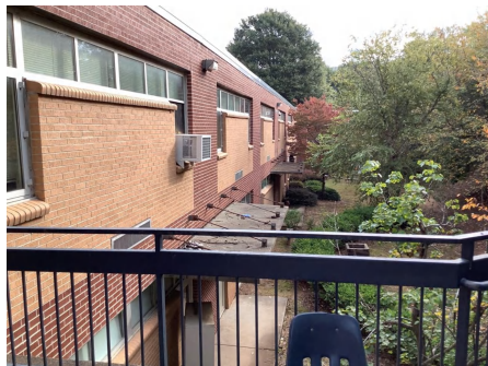
4). Southwest Elevation - Dec 11, 2019
