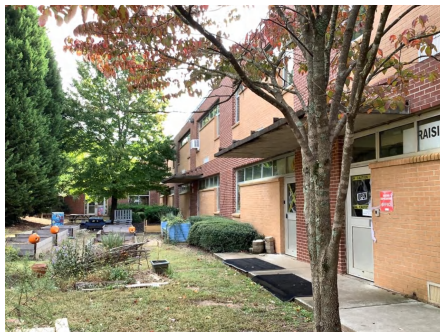
3). Southwest Elevation - Dec 11, 2019
