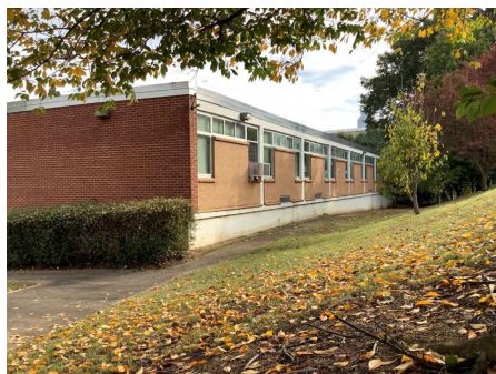
4). Southwest Elevation - Dec 11, 2019
